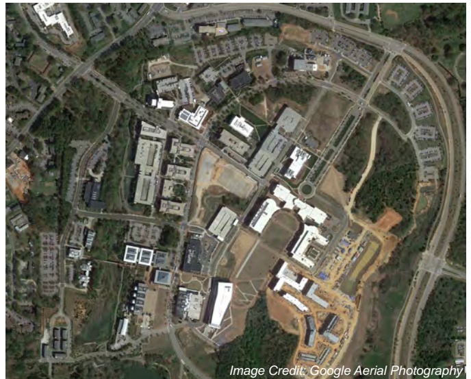
Image Credit: Google Aerial Photography
